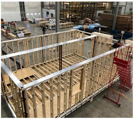
The internal wall sub face is added, enabling first fix electrical and plumbing to be installed. This process takes only hours as the building is in skeleton form with free open access to all areas.
